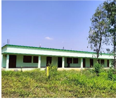
Well ventilated building structure
